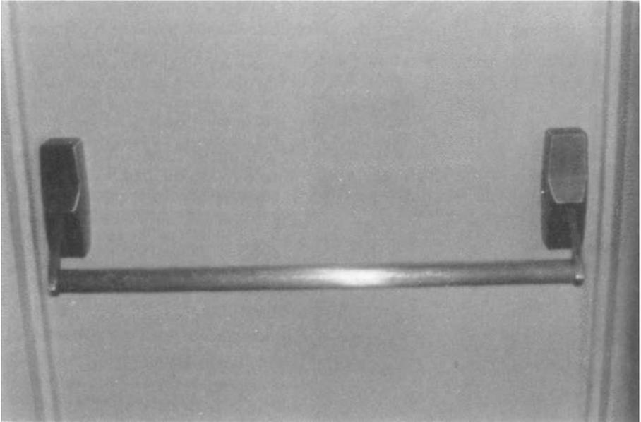
4.3 Doors in Two Commercial Buildings. Pushing the bar opens the door, but on which side do you push? Bar *A* (above) hides the signal, making it impossible to know on which side to push. A frustrating door. Bar *B* (below) has a flat plate mounted on the side that is to be pushed; this is a naturally interpreted signal. A nice design, no frustration for the user.
