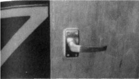
The handle depicted at the left shows inappropriate signals. This form of handle clearly marks grasp, twist, or pull—except that this particular door slides: a classic case of inappropriate design.
