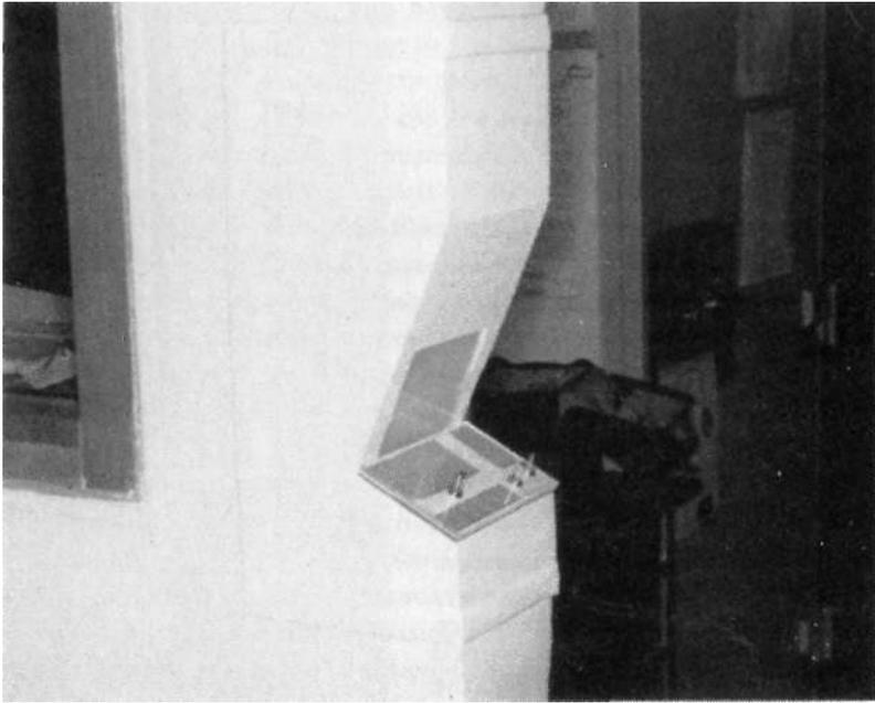
4.8 The original layout of switches in my laboratory had the light switches scattered. We put all the switches in one convenient location, arranged on a floor plan of the laboratory. (The switch panel was constructed by David Wargo.)
